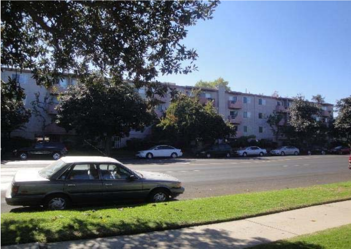
VIEW OF SITE FROM NORTH
