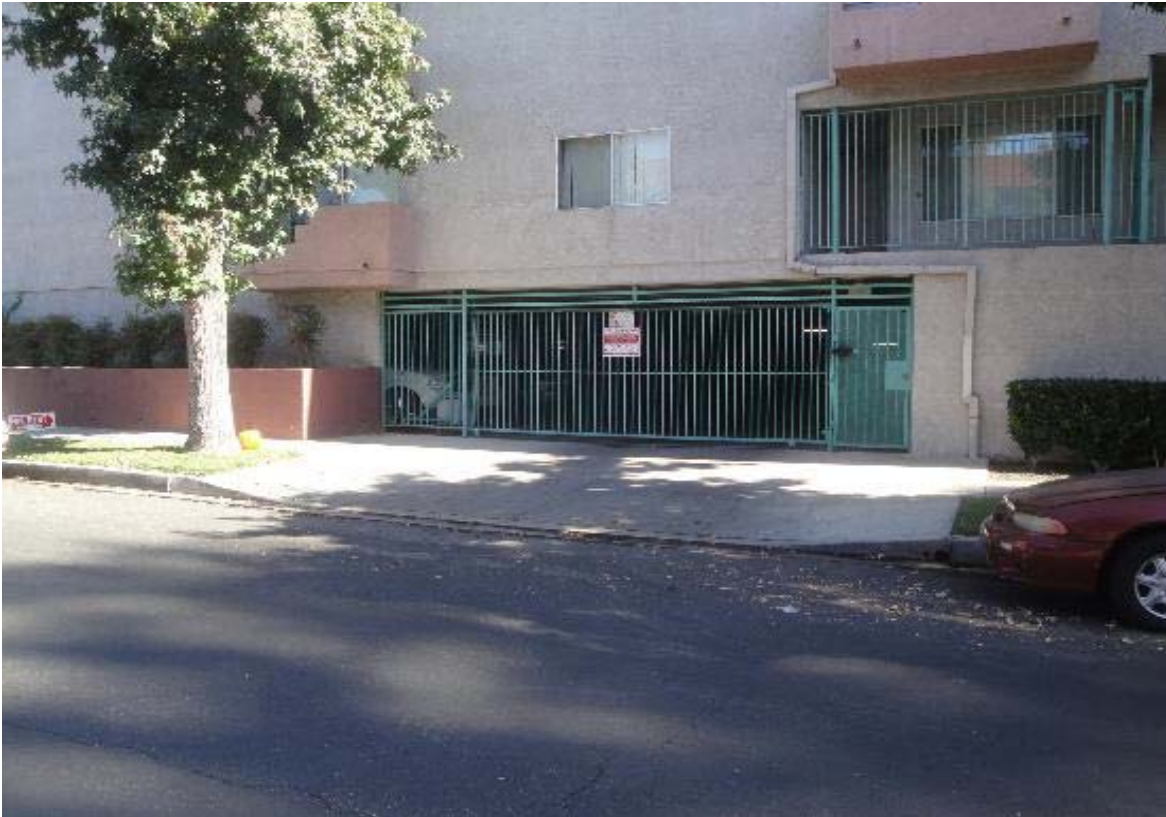
VIEW OF SITE ACCESS
