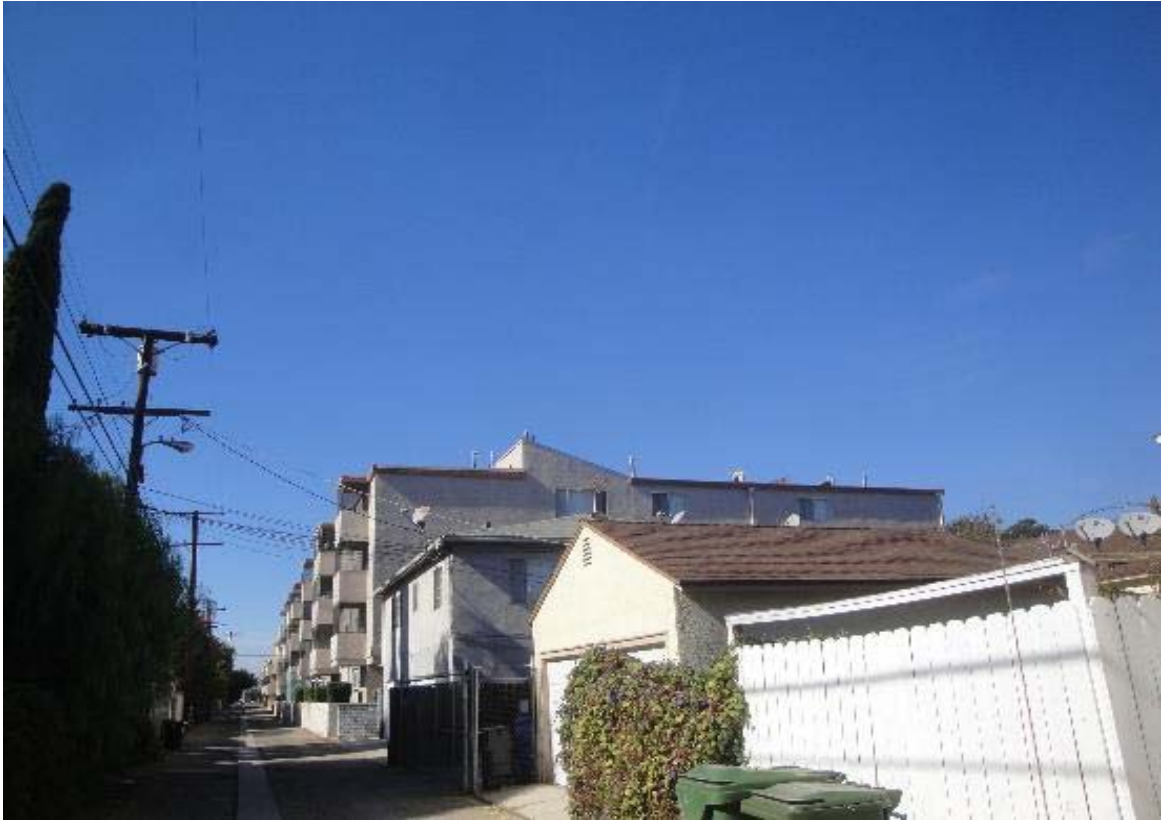
VIEW OF SITE FROM EAST
